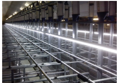
Renovated stables in Holland
