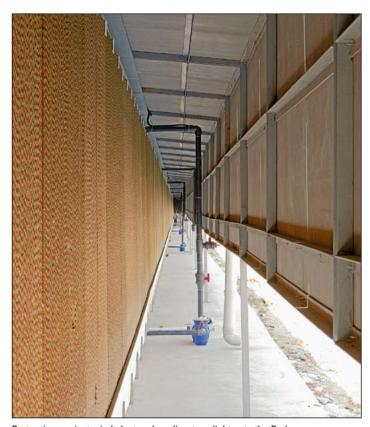
Protection against wind, dust and no direct sunlight onto the Pad
