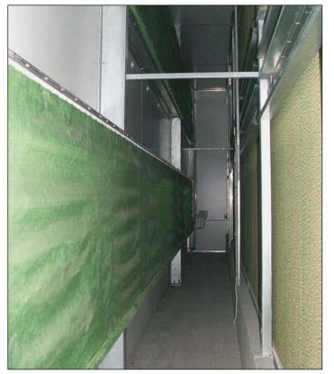
Tunnel inlet with roller curtain
