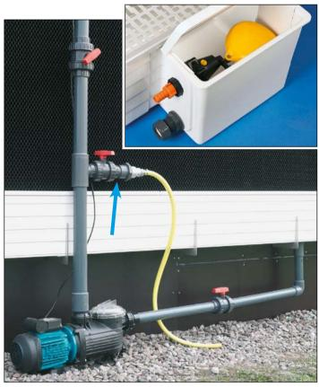
Centrifugal pump incl. filter and bleed-off
