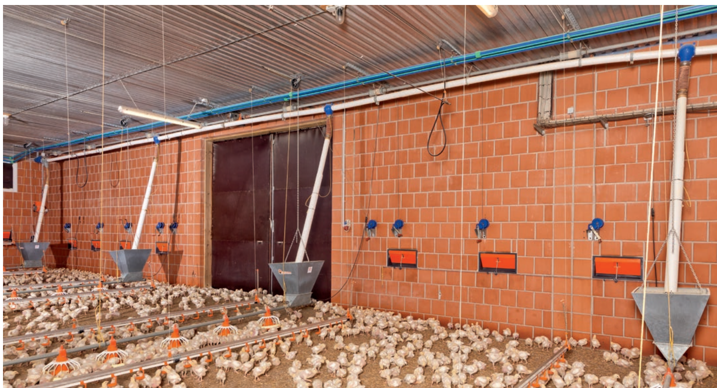
Use of cable winches for optimum height adjustment of the drinker lines in relation with the birds' age
