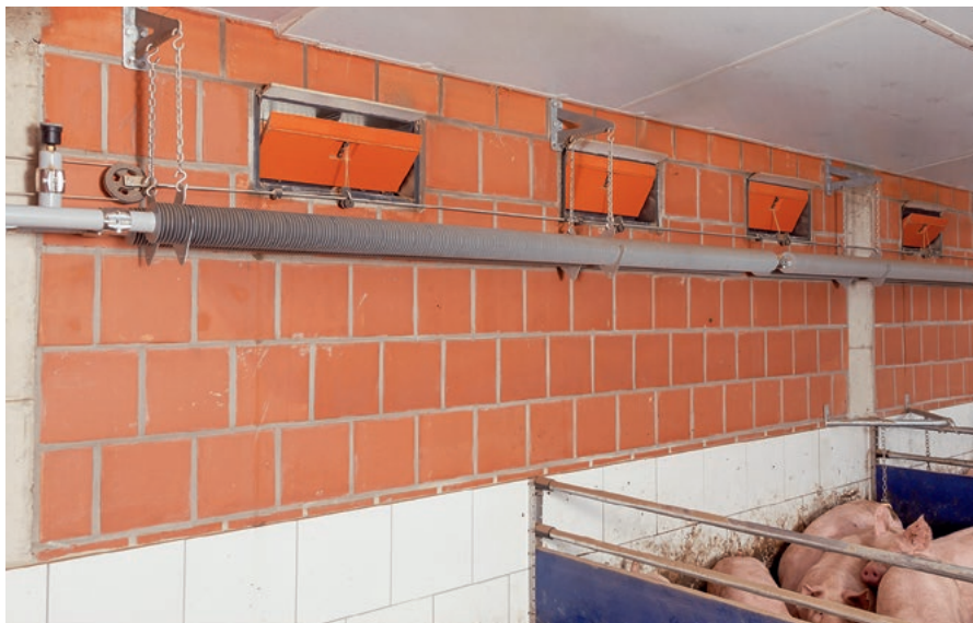
Aluminium fin heater as a full-space heating system – ideal in combination with fresh air inlets
